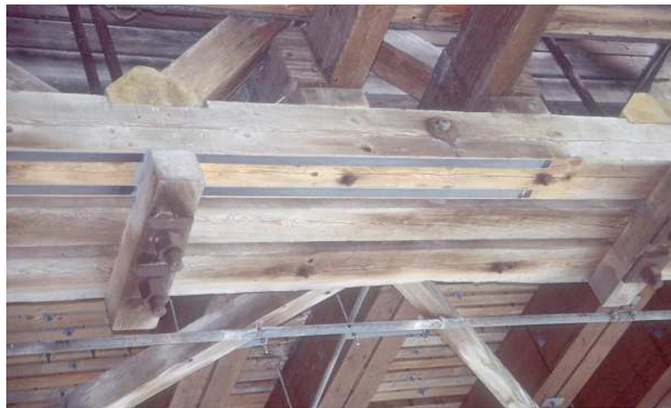
Fig. 1. Restrengthening of bottom chords of the timber bridge (Steiger 1999)
