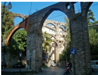
The “Devil’s bridge” and its pointed arch.
